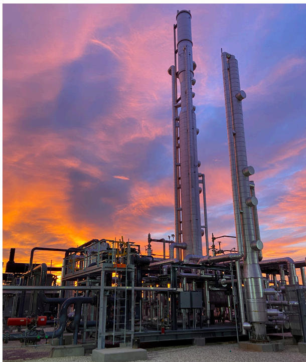
Figure 1. 50 million ft 3 /d NiTech IV two-column cryogenic NRU in West Texas, US.
